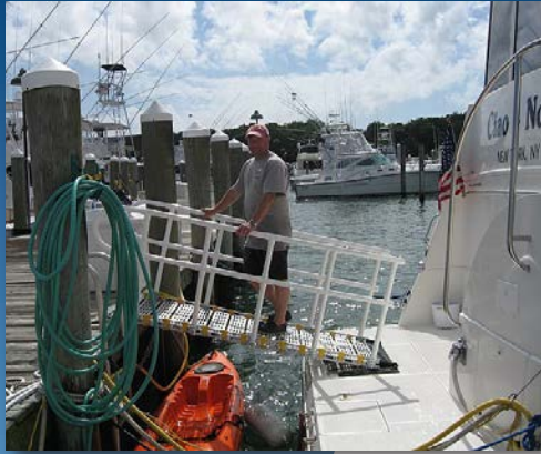
Dock to yacht or watercraft. Ramp rises and falls with water level.
